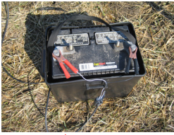
Power cable connected to battery
